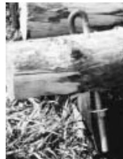
*A simple pass-through for an interior pole: a piece of threaded rod with a hook bent into one end. The hook closes against the pole as the nut is tightened.*
